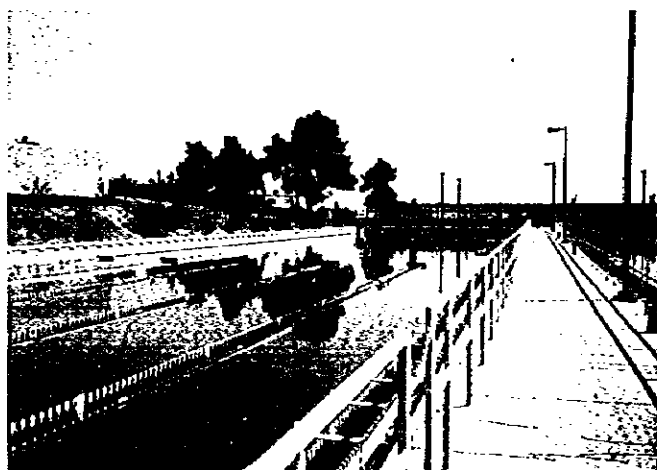
沈でん池及び薬品注入棟 Sedimentation Basin and Chemical Building
