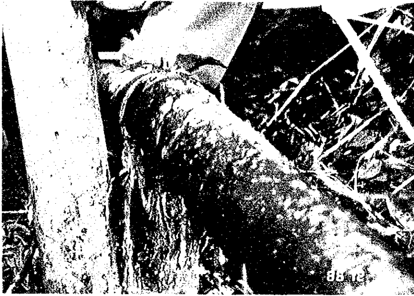
No.6 Damaged Existing Pipe
