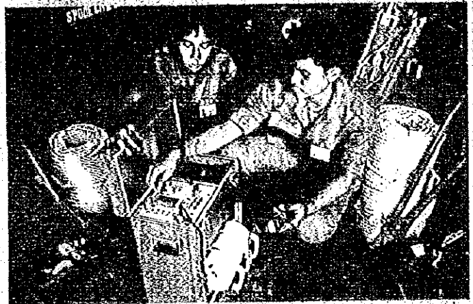
Trapped Person Locator - Detects life trapped under debris.
