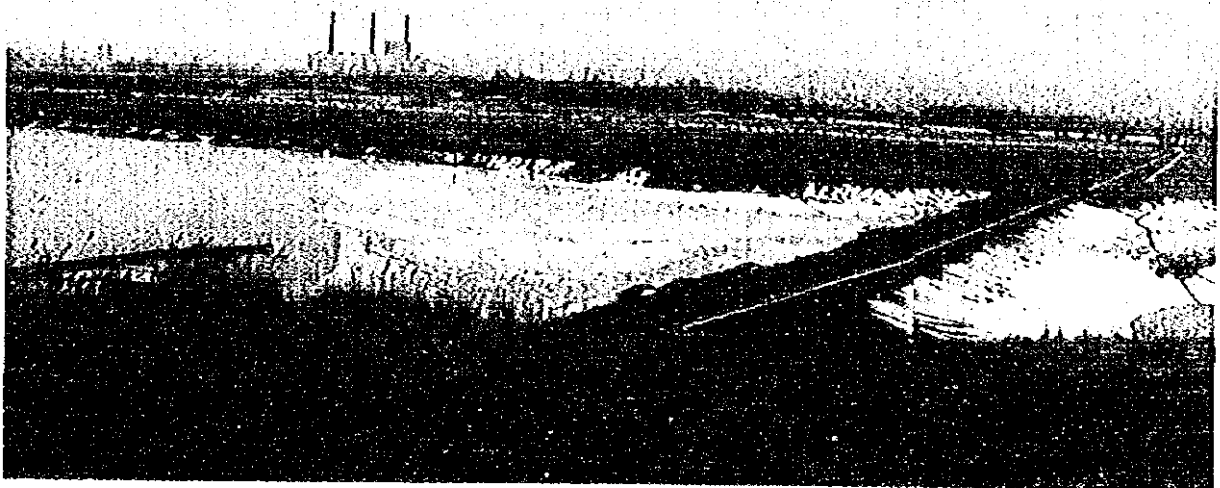
Thick Slurry Pipeline and Slag Area
