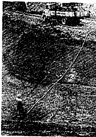
Diagram 3-23 Seeding Work with Pump (Spraying Work)
