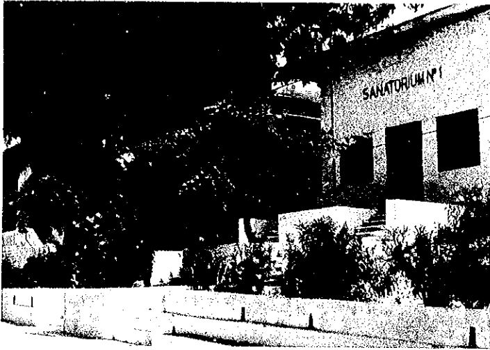
SANATORIUM DE PORT-AU-PRINCE
