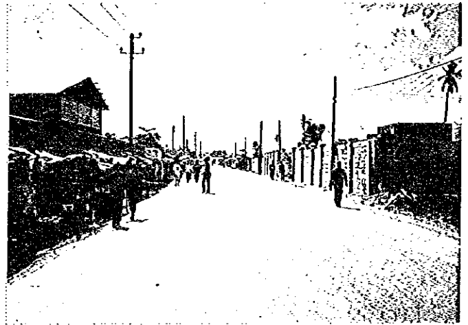
The condition of Vingunguti Road near Nyerere Road.
