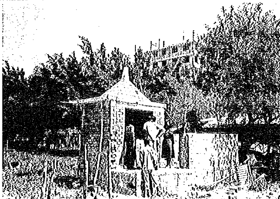
Picture : The Incinerator in Mission Mikocheni Hospital under construction in August 1996
