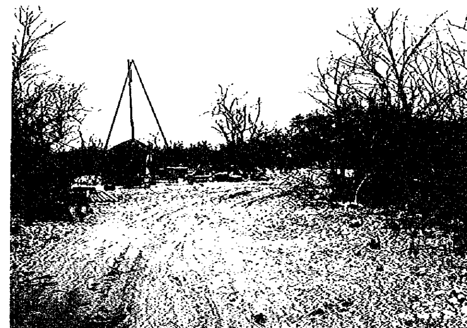
Drilling of MJNM-1 by L-38
