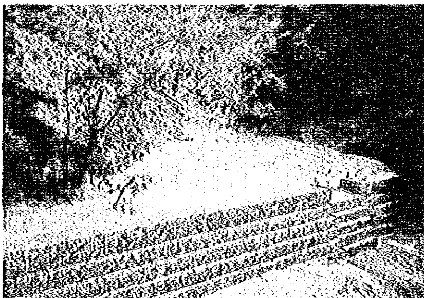
Plate 4. Photo : DPTC Gabion Check Dam for Toe Loading at 62 km. along Charali-Ham Road.
