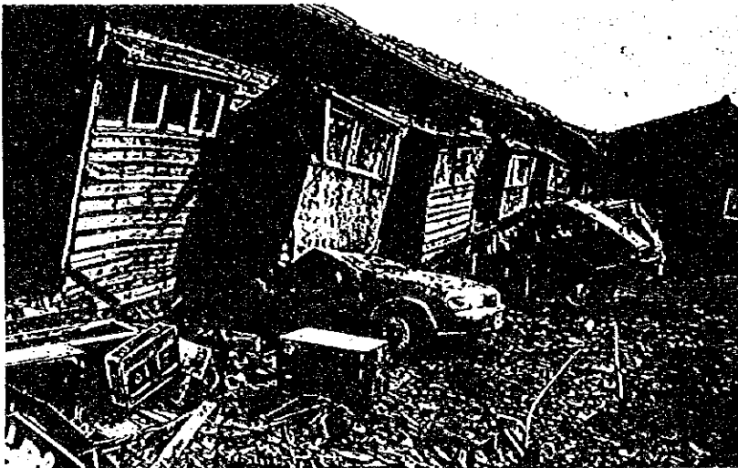
Offering little resistance, more than 50,000 wooden houses collapsed in the quake.
