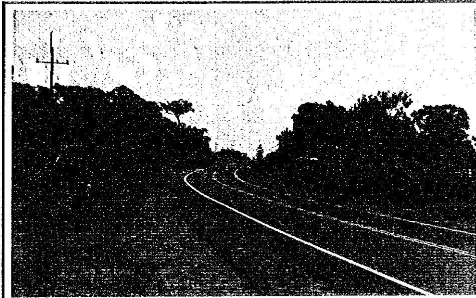
Photo-7 Junction point with Acahay - La Colmena road.
