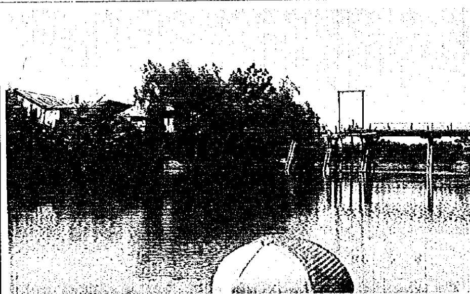
Photo-5 Existing wood bridge on Tebicuary-mi River. (Bridge length = 70m)
