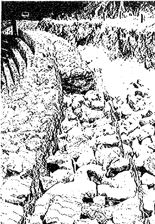
Photo 1.5.9 Example of Gabion propwall construction under People's participation. (Daman, Tribhuvan Highway, Daman VDC, Makwanpur).
