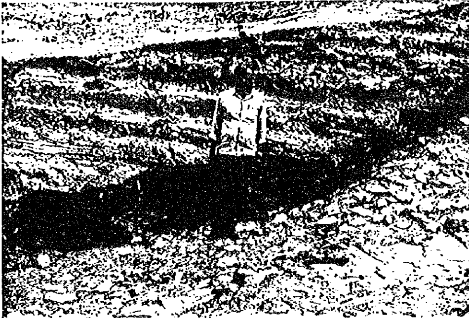
Photograph Showing Sediment Deposited in the Kulekhani Reservoir near the Chitlang Khola Confluence (the gravel of road pavement is also clearly seen)
