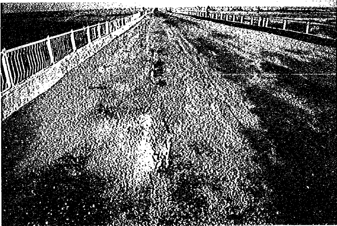
Photo 12 : Bridge No. 28 (Kzyl-Orda Border to Irgiz)
