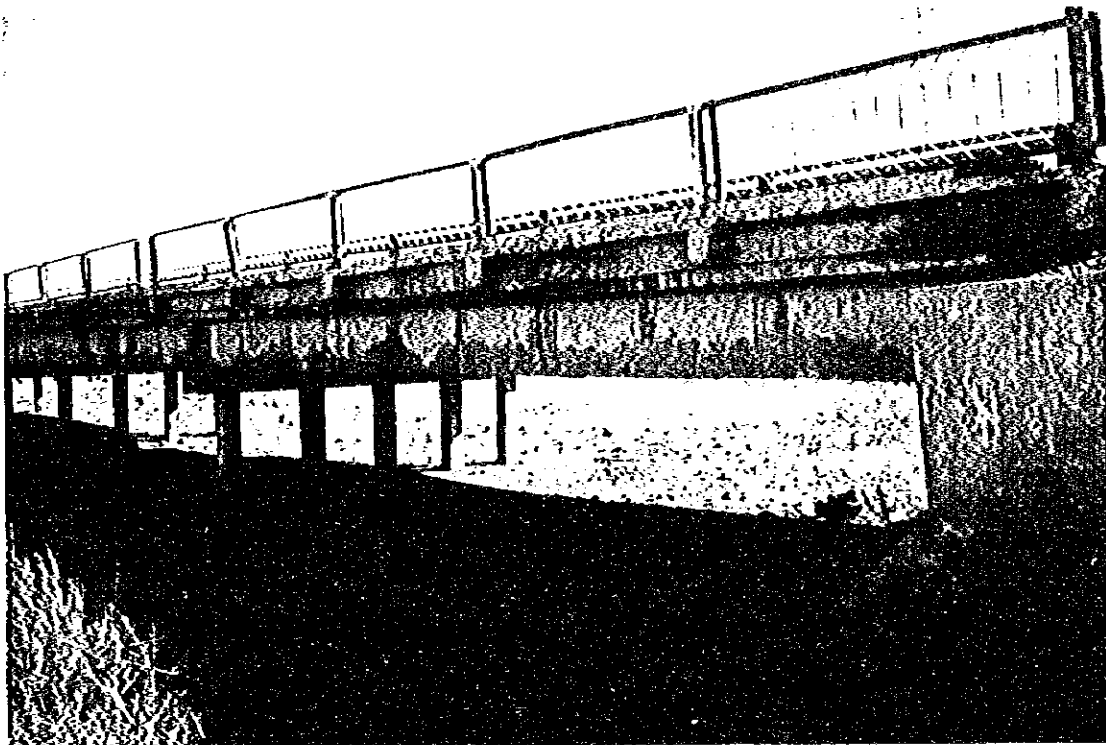
Photo 13 : Bridge No. 2 (Atyrau to Mahambet)
