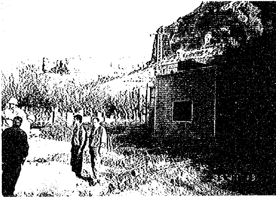
Well bored near a Generator House
