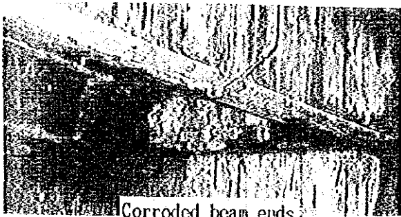
Corroded beam ends
