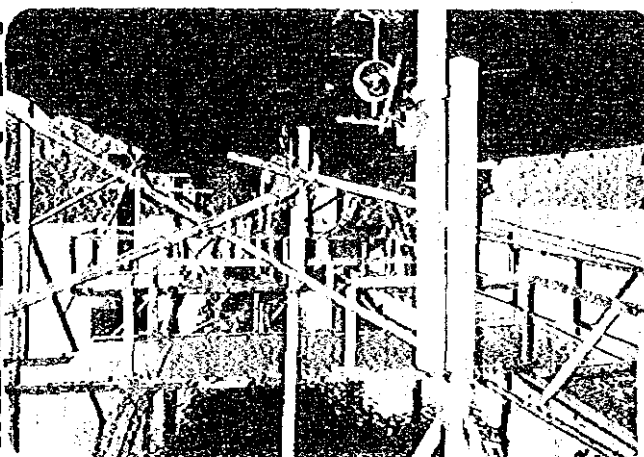
Scaffolding for loading test Ser No. 59
