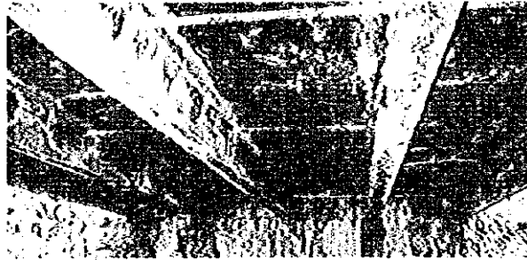
Free Lime from Buckle Plate Slab (BUC)
