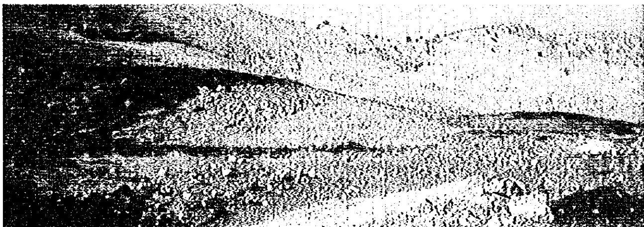
View of landfill. Cover soil is not implemented, and open dumping is executed.
