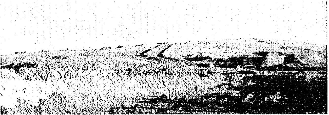
View of sprinkling cover soil with supernatant of treated night soil.
