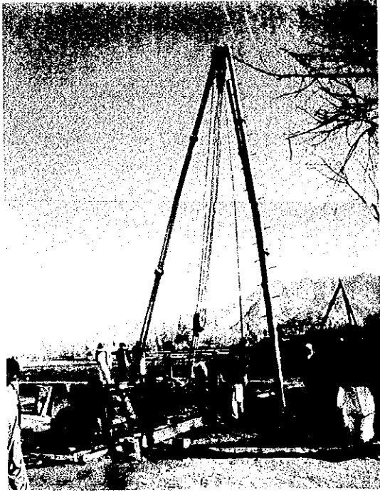
⑦ Drilling Works by Hand Plant (Dir District)
