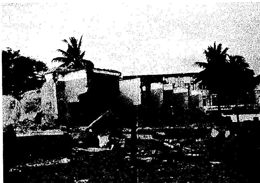
A Building Under Demolition On The Site 解体中
