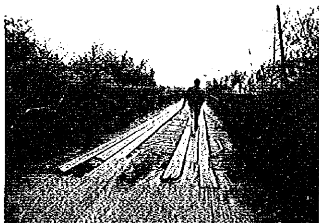
写真-53 Tebicuary Mi~Tebicuary間道路に架かるペイリー橋。橋長40m。
