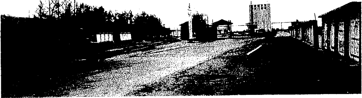
A truck scale house is in front and a high building in the back is a feed mill. Access road to front gate is well maintained. (Harhorin)
