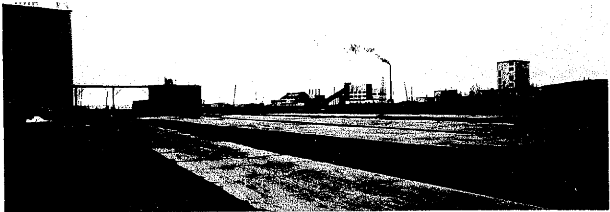
The site reserved for construction of grain storage facility at Harhorin. Presently used for open yard piling of the wheat that could not be stored in existing warehouse.
