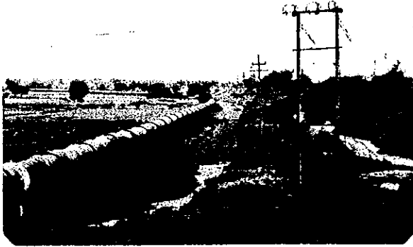
The water main on the upstream side along the existing approach road
