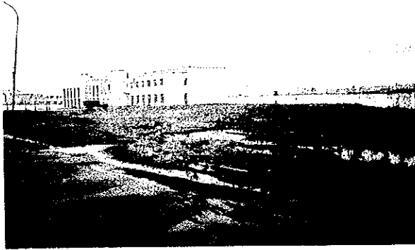
The Project site (approximately 4 ha) is located within the sub-depot of the Passenger Transport Bus-1 Company, where sufficient space is available. The building in the back is the welfare facility.
