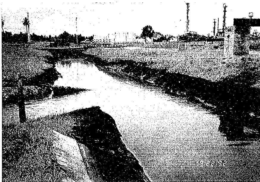
Outlet stream from Nos. 3 and 4 API separators. The mark of black oil on the banks suggests incidental oil spills.
