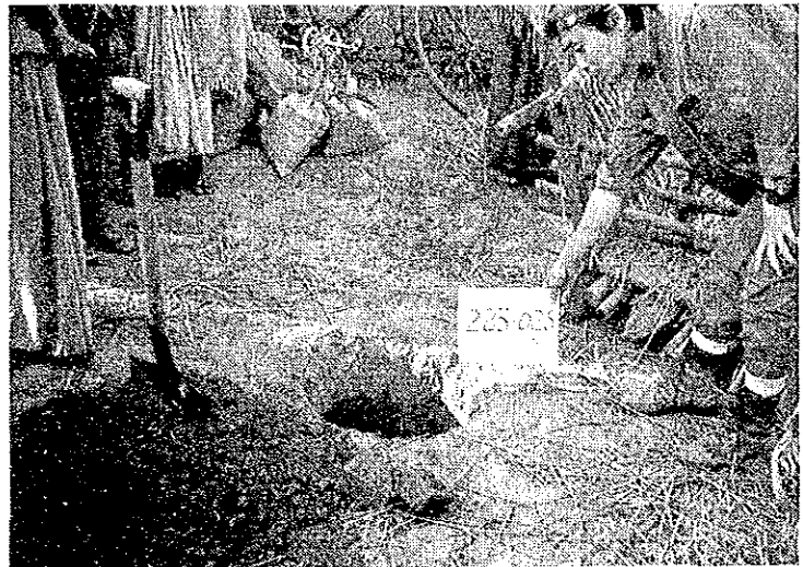
Bench Mark burried under ground.
