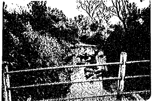
LB Feeder Canal
