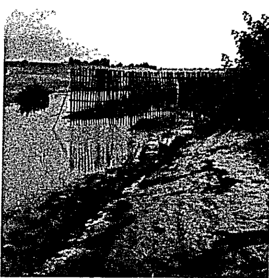
The scene of a simple bank protection palisade.
