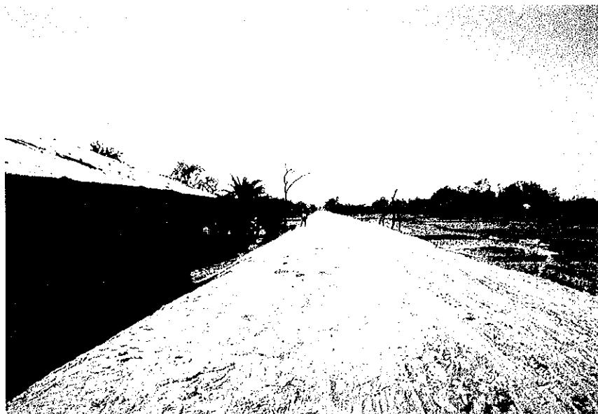
Road Conditions near the Site
