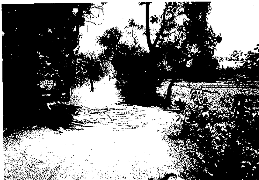
Road Conditions near the Site
