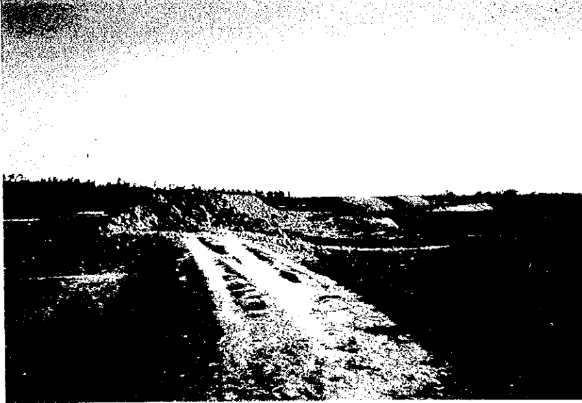
Current Conditions near the Site (Embankment being constructed)
