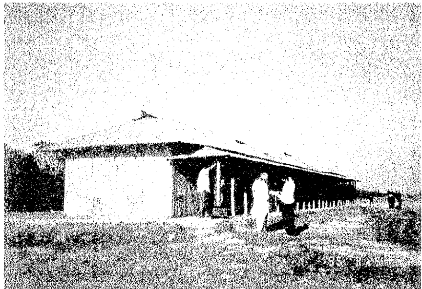
Overall View of the School Building
