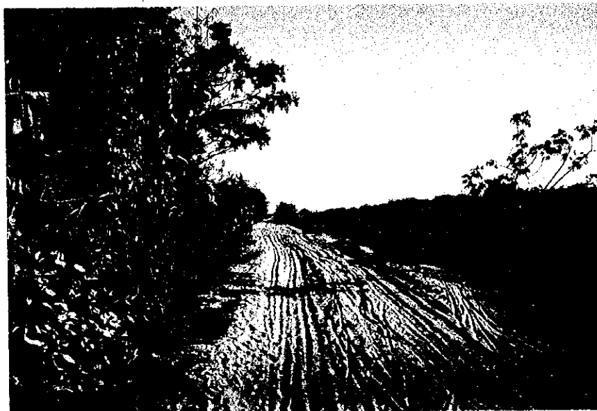
Road Conditions near the Site
