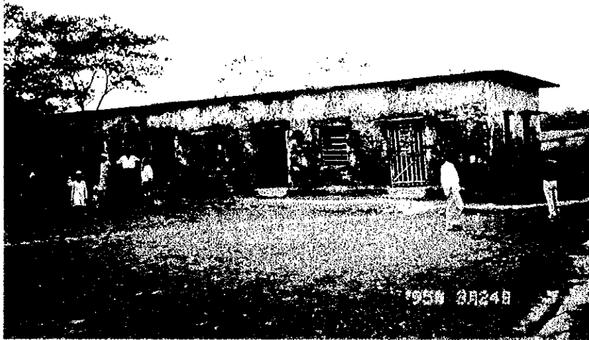
Overall View of the School Site
