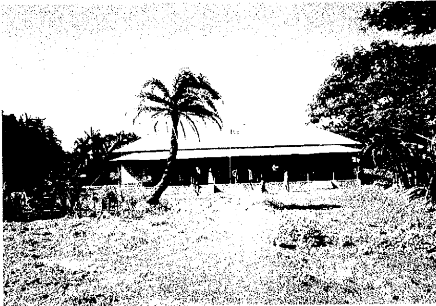
Overall View of the School Site
