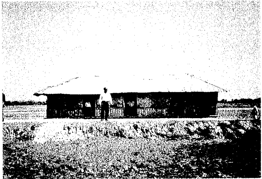
Overall View of the School Building
