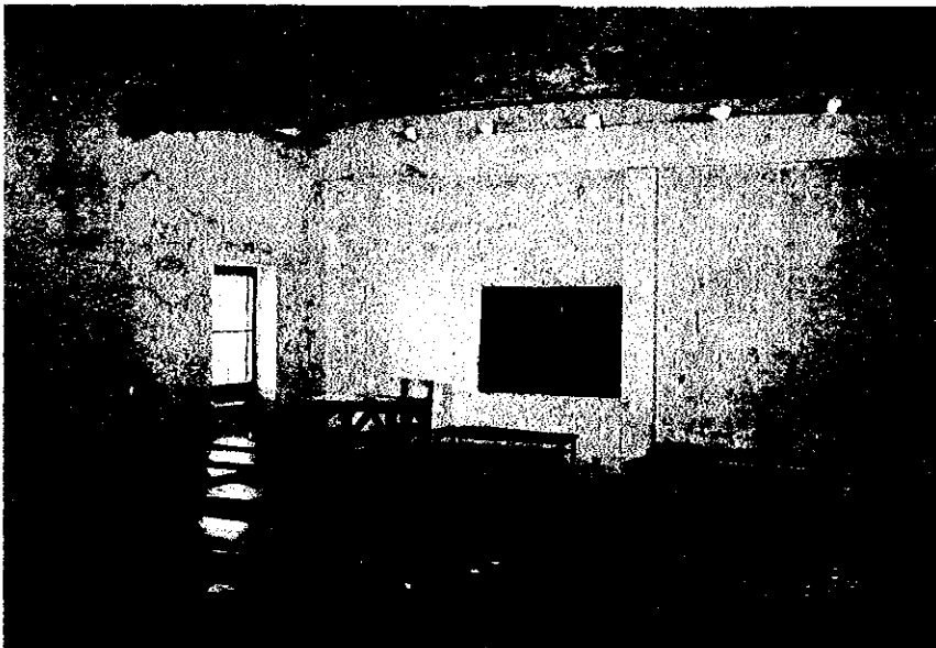
Current Conditions of A Classroom
