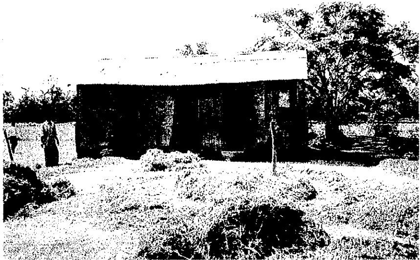
Overall view of the School Building
