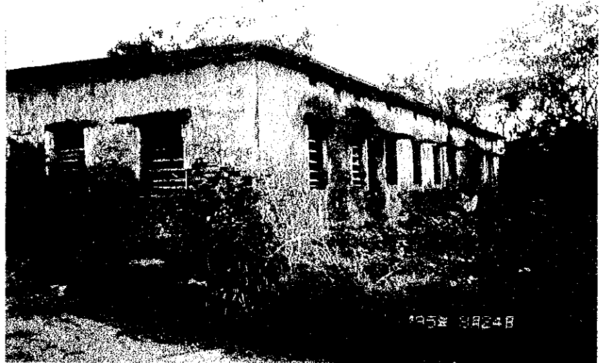
View of the School Building
