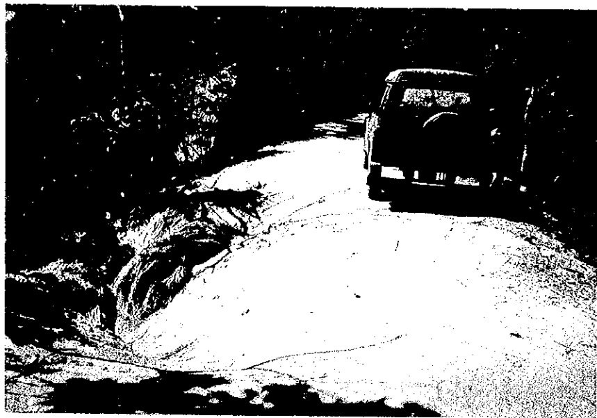
Road Conditions near the Site
