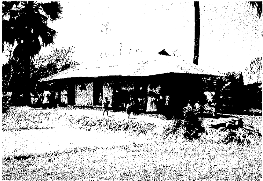
Overall View of the School Building
