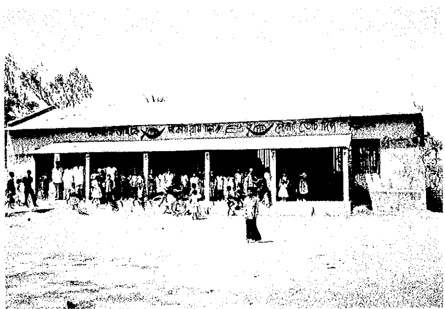
Overall View of the School Building
