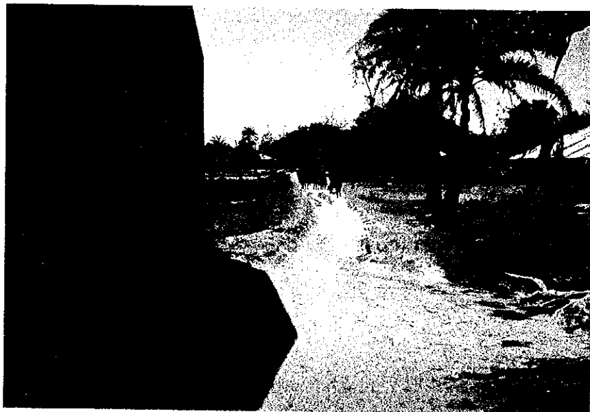
Road Conditions near the Site
