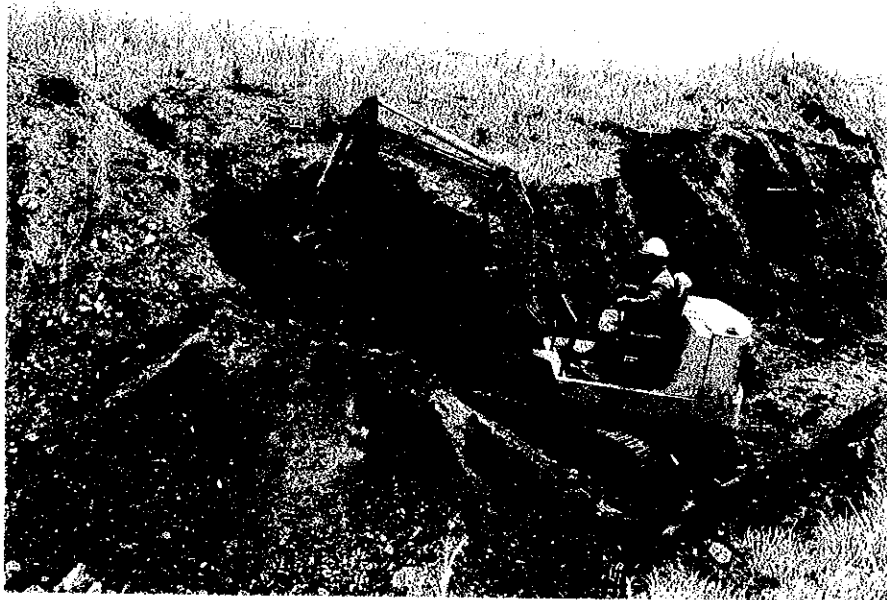
Trench excavation by Back Hoe
