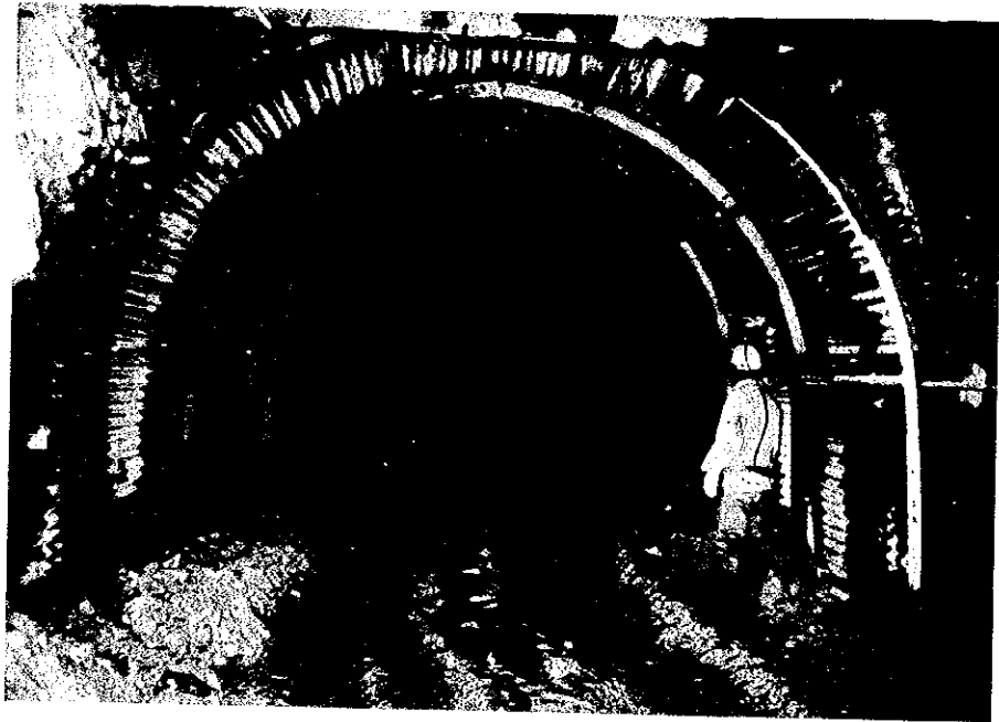
General view of No.4 Waste pit
