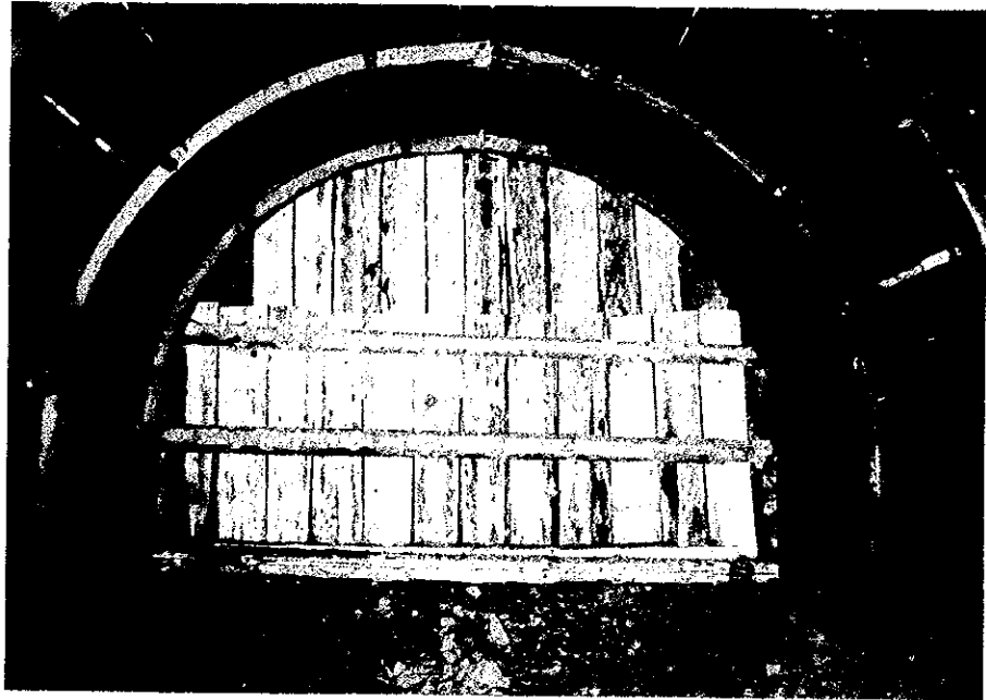
Face of No.4 Waste pit
