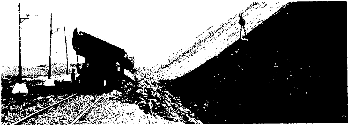
Dumping Overburden from Wagons at Overburden Dump
