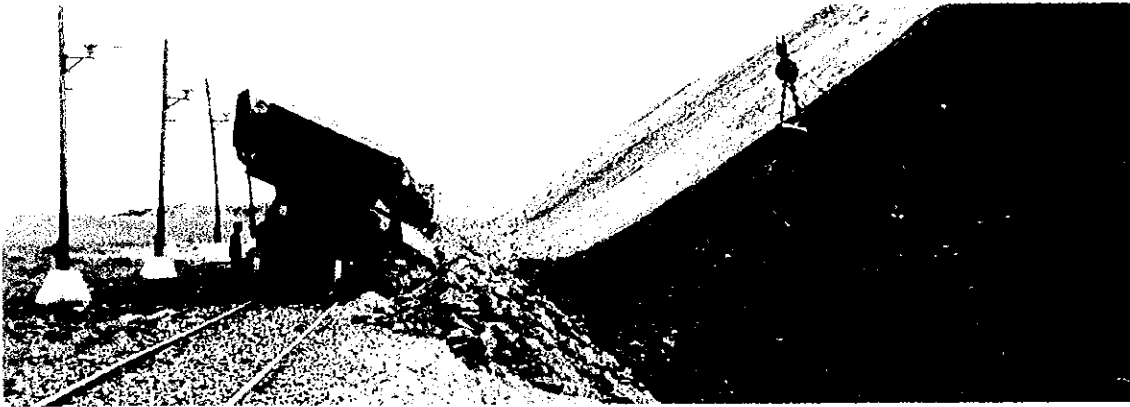
Dumping Overburden from Wagons at Overburden Dump
