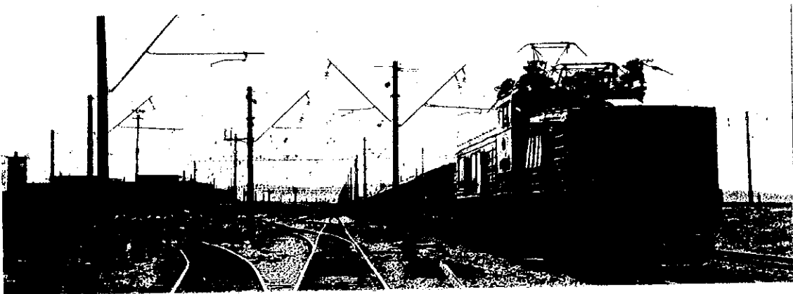
Transportation of Overburden by Railway System
