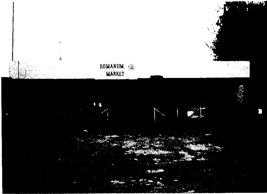
Fish market in Weno (Local office of a cooperative from an island inside the Chuuk Lagoon).
