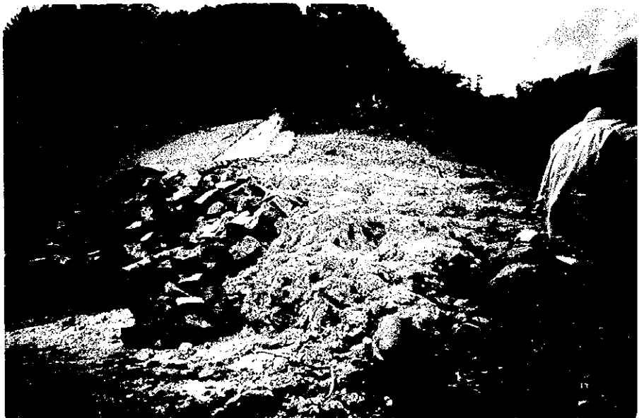
13. Land Slide Occuring around Inlet Channel of Intake Structure (1/2)
