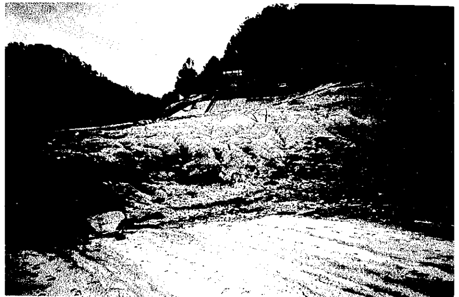
14. Land Slide Occuring around Inlet Channel of Intake Structure (2/2)
