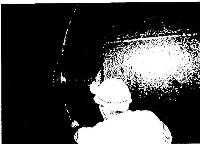
5. Leakage from No.1 butterfly valve (No leakage)
