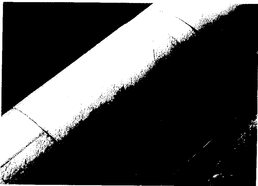
E-4. Butt welding joint type double layer penstock at No.82 unit pipe
