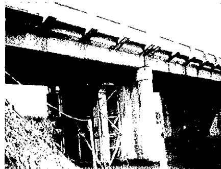
LIBOGANON BRIDGE: SUFFERING FROM PIER SETTLEMENT
