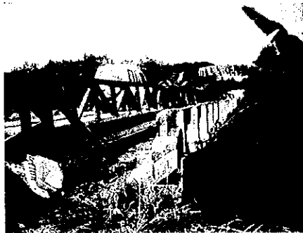
PANAYTAY BRIDGE: SUPERSTRUCTURE NO LONGER FUNCTIONING
