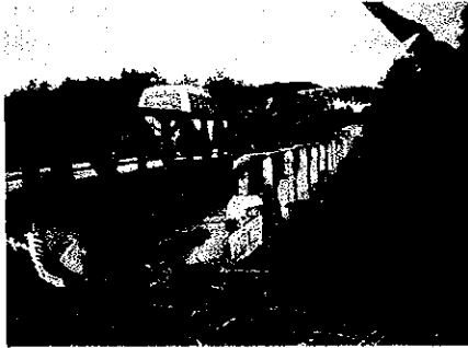
PANAYTAY BRIDGE: SUPERSTRUCTURE NO LONGER FUNCTIONING
