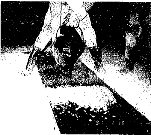
Repairs for Expansion Joints
