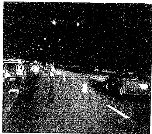
Traffic Regulations for Maintenance Work (2)
