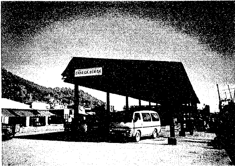
Photo - 10 "Ben Da" Principal Fishing Port within Vung Tau City There is a landing dock and a fish handling area. However, comparing with fishing fleet, facilities on land are too short. There are some small workshops and fuel supply facilities.
