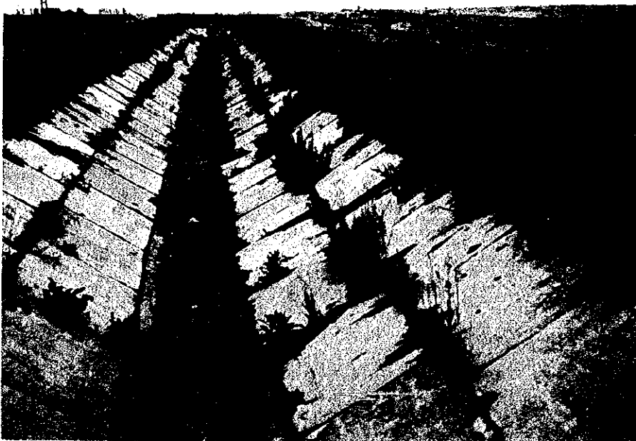
10. Completed Section of Distribution Canal Damages and sliding of panel and soil-inflow through the joints are seen in many sites.
