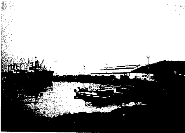
Wharf DII of Port of Panjang, Bandar Lampung
