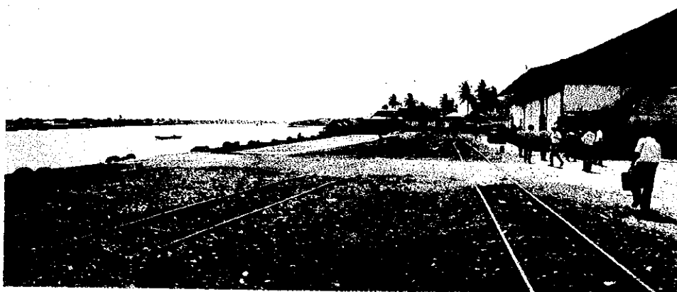
Kertapati Dry Port along Musi River. Palembang Port is located opposite side of the River. (South Sumatra)
