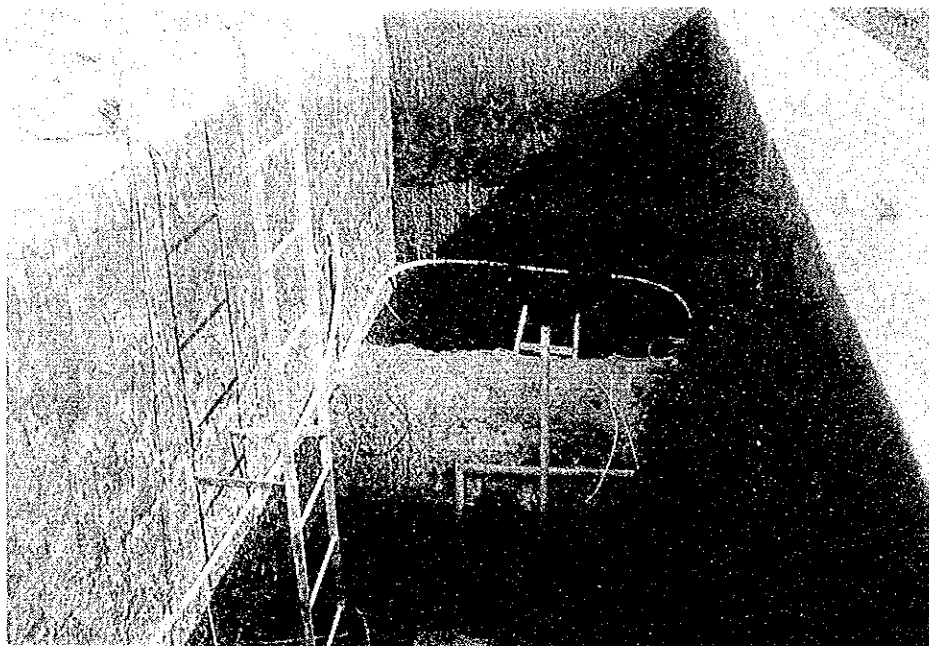
Photograph 2 - 13 Distribution water flow meter (for mains pipe) detector unit pit
