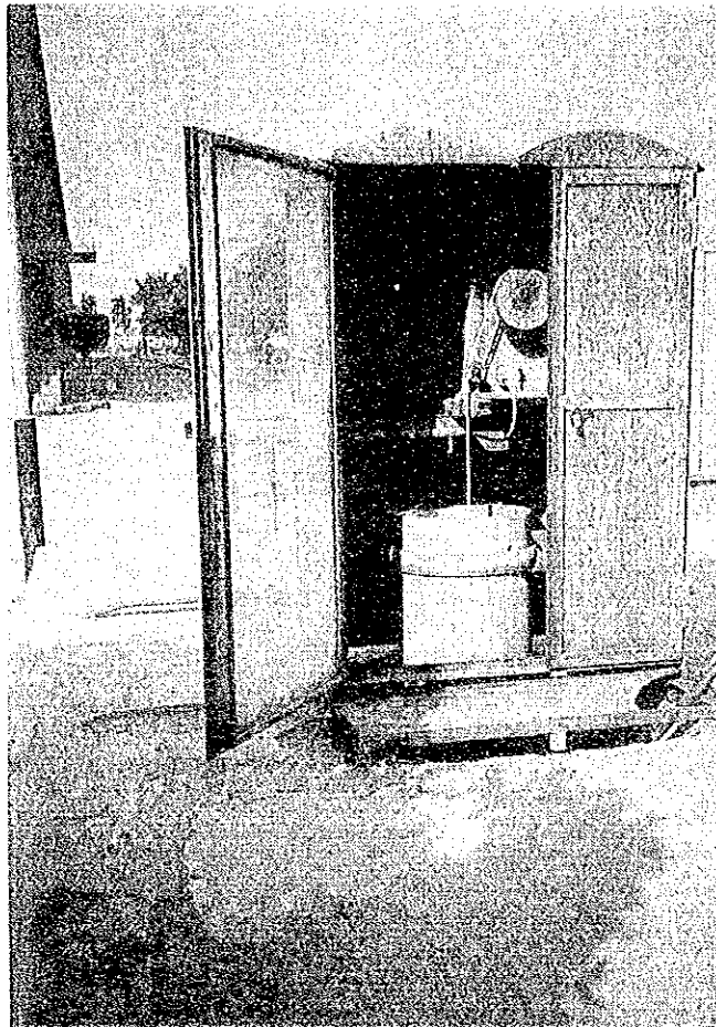
Photograph 2 - 12 Water treatment plant water level meter transmitter unit
