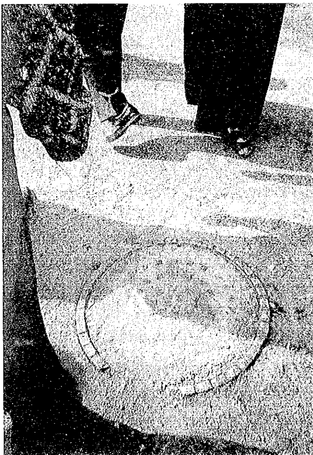
Photograph 3-3 Manhole of the sewer receiving waste water from the shared used tap shown in the photograph above
