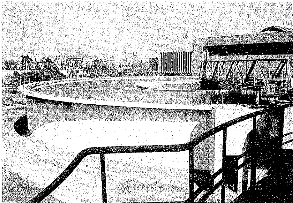
Photograph 2 - 16 Sedimentation basin (there is no structural problem)
