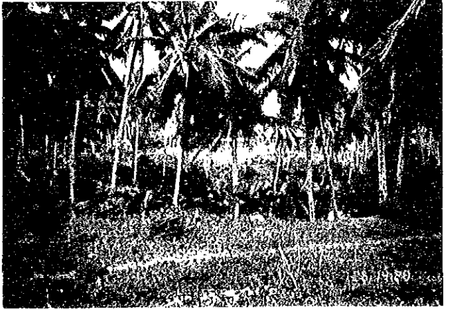
橋梁位置 : Km. 1649+210 Davao Oriental-Surigao del Sur, Coastal Road Manay, Davao Oriental
