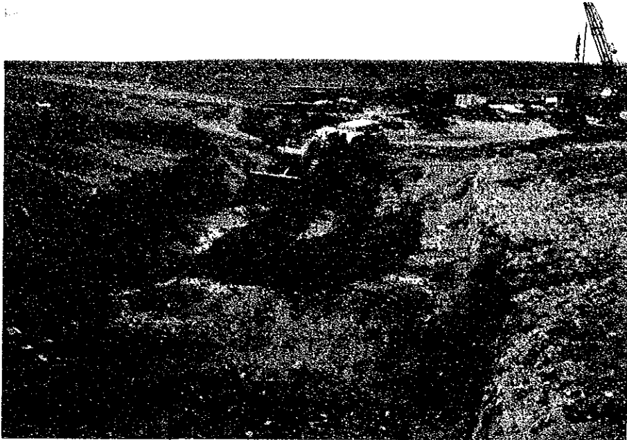
Excavation of mine portal
