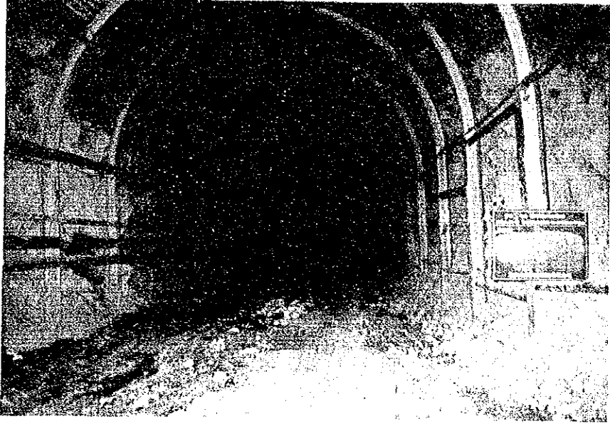
Inclined shaft (type 3)
