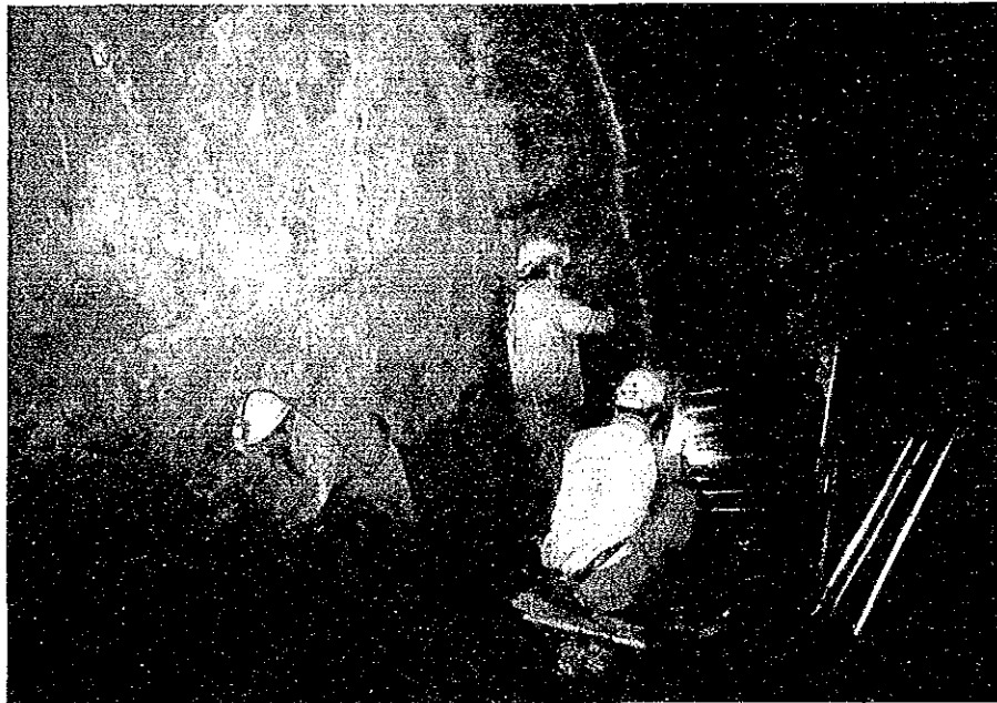
Timbering (steel board)
