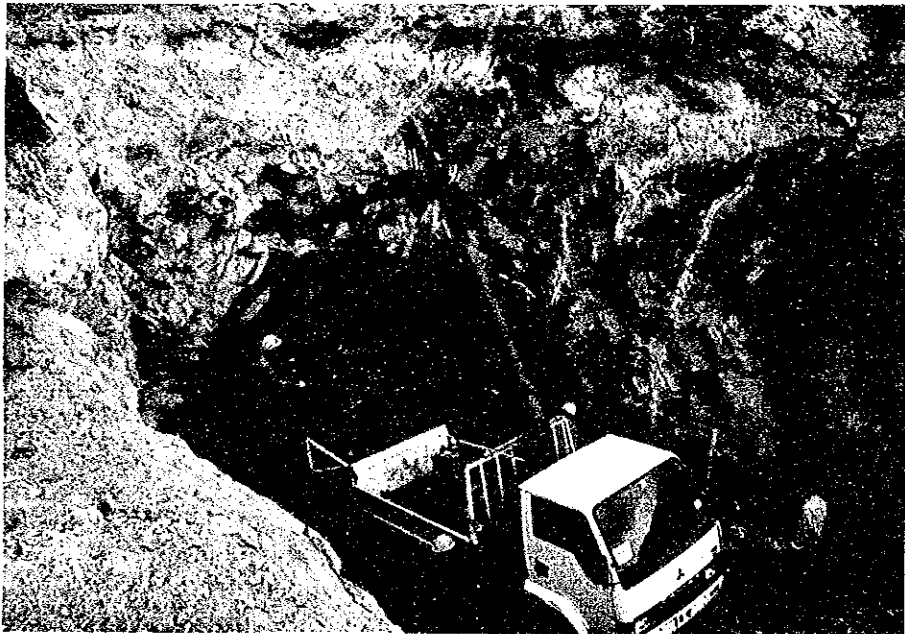
Construction of mine portal (frame)
