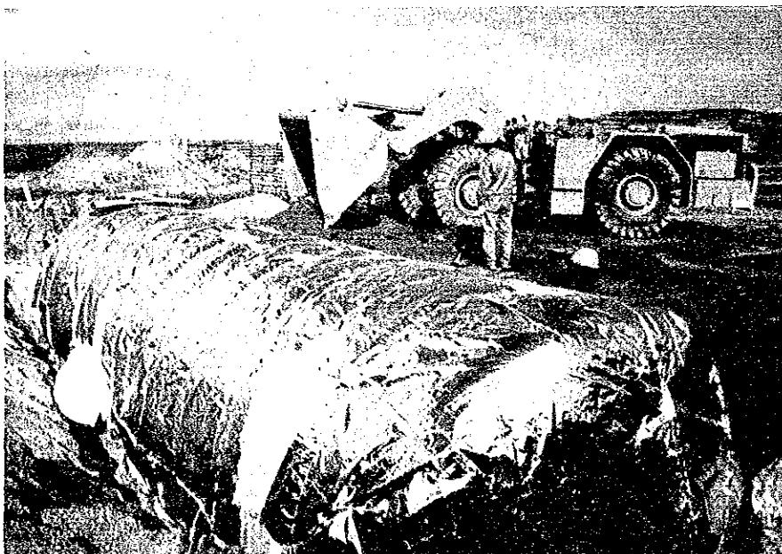
Establishment of water tank
