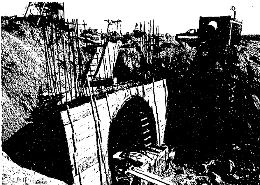
Construction of mine portal (assemble)
