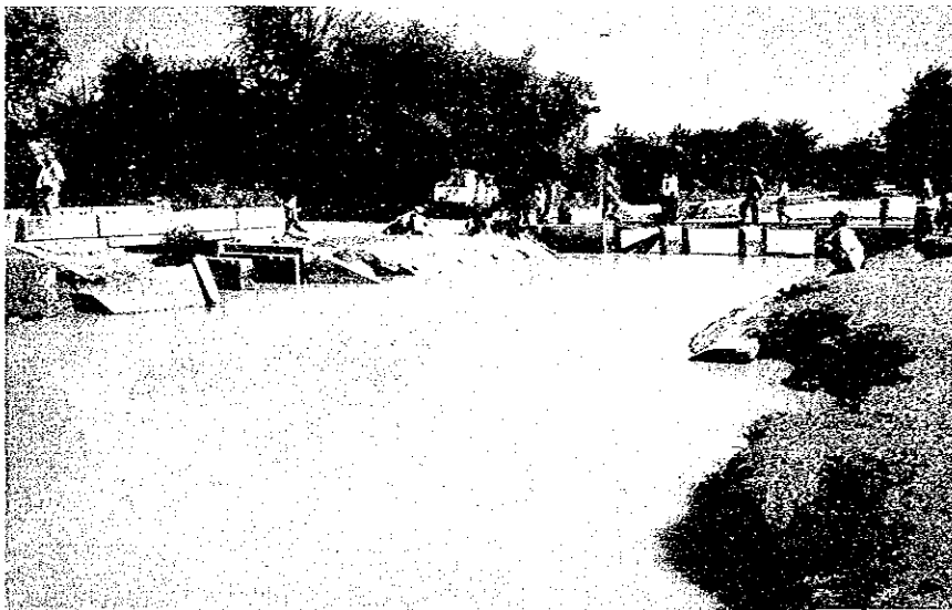
Intake from Bovel Irrigation Canal to the Center Farm
